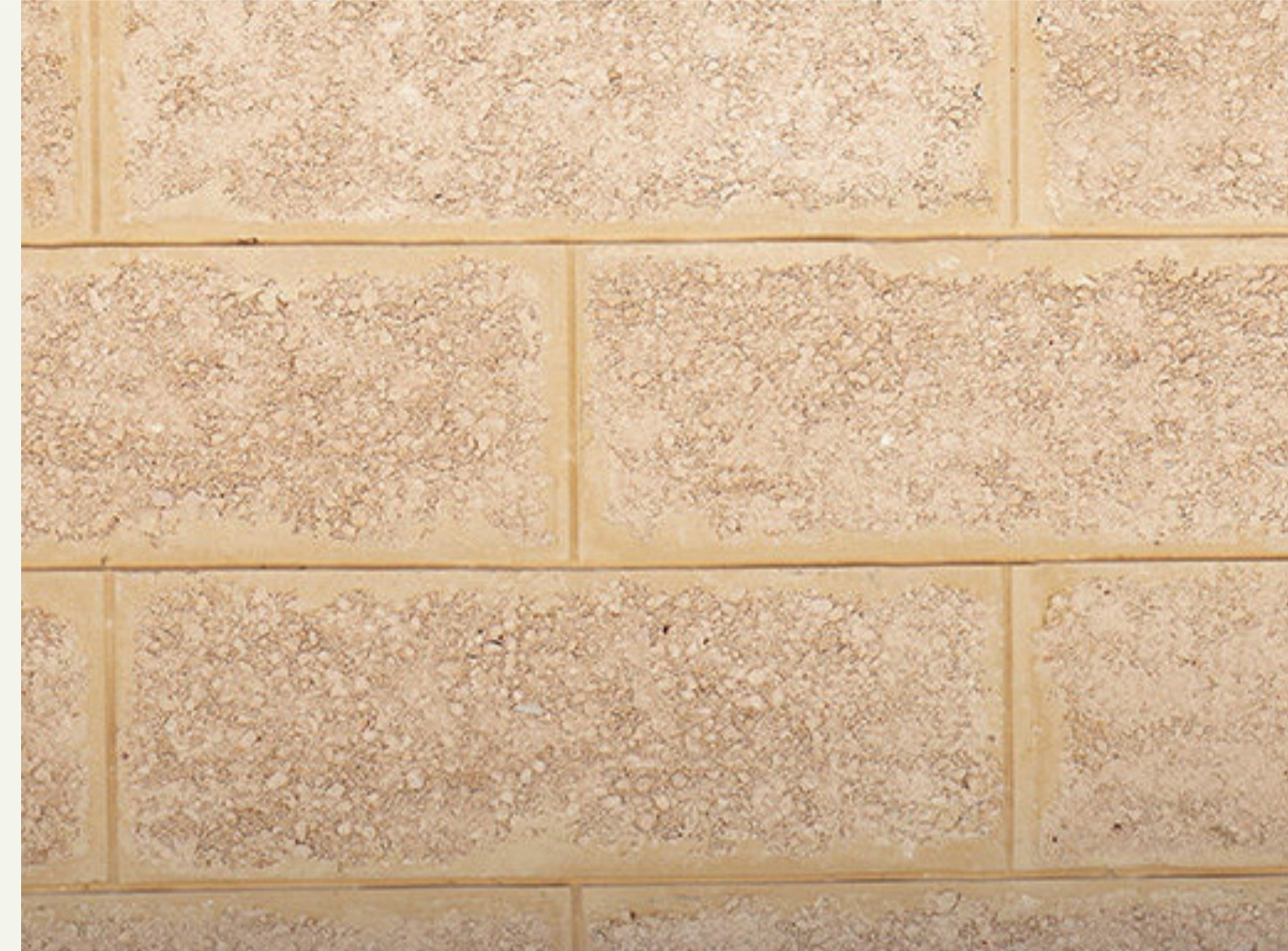
LIMESTONE RETAINING WALLS
