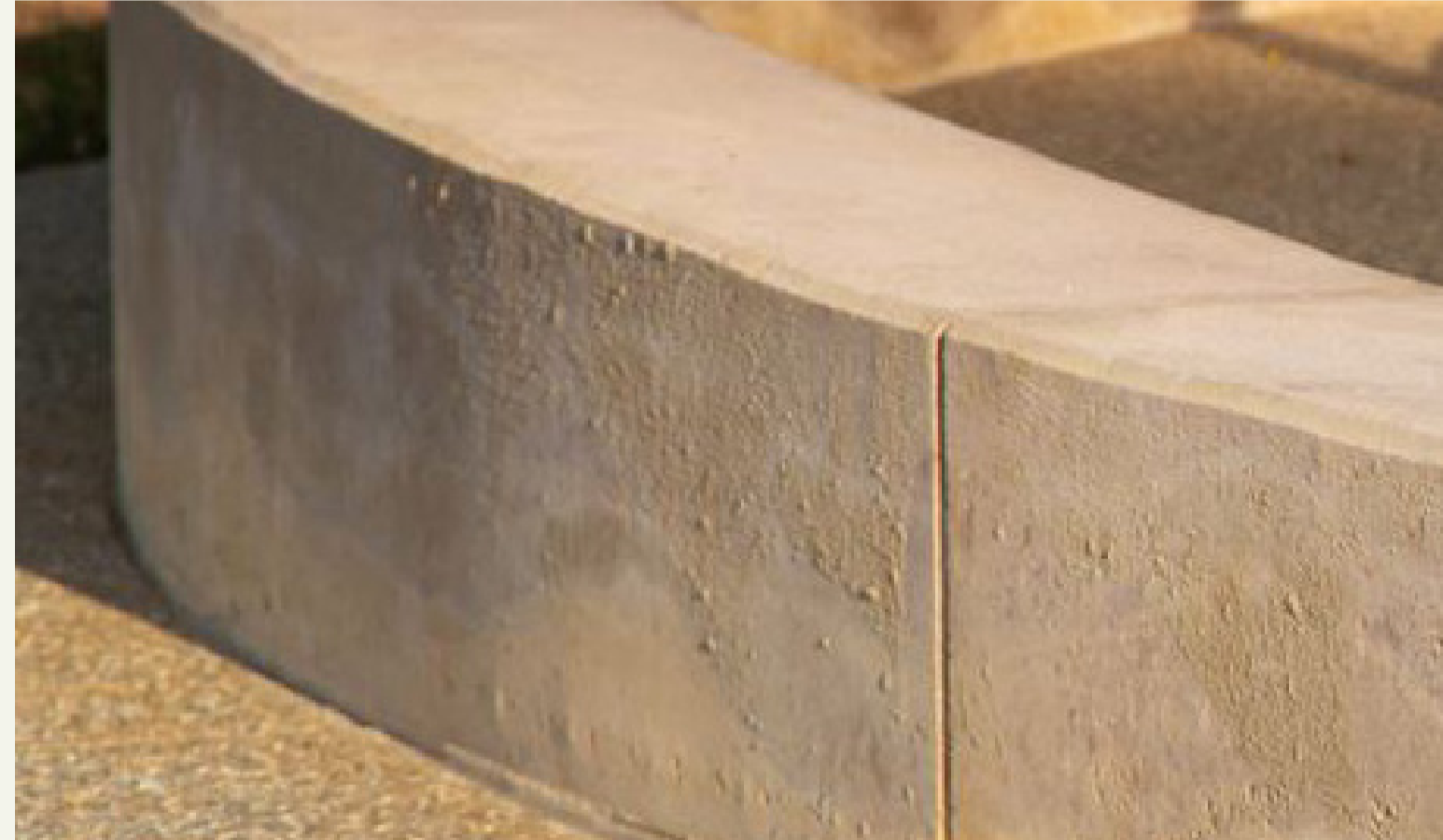
RAMMED EARTH WALL
